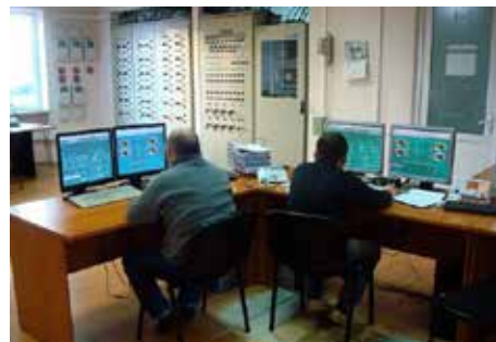
Dispatch room, two workstations equipped with double screens, Switchboard with glass window and TC 700 control unit supplied by Teco.
