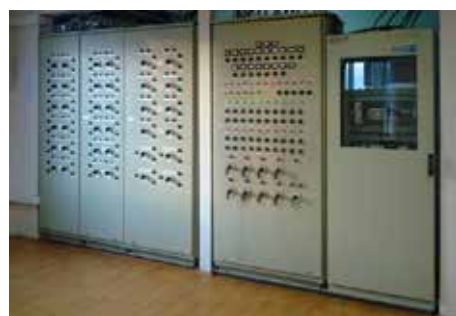
Typical set of 2 switchboards for 4 tanks with the relevant group of automatically controlled valves.
